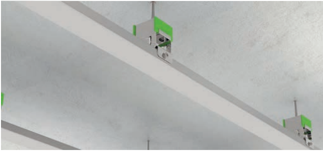
9.- Acoustic hangers and profiles fixed.
