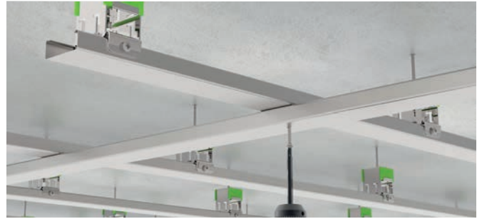
10.- Place transverse profiles in position.
