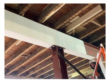
"The tested and smart solutions with PROMATECT®-100 boards with a single sheet layer under wooden floors are ideal. It makes huge savings in transport movements and installation costs."
